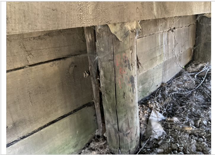
Bent 8 pile 2 is hollow and split 2022 picture
