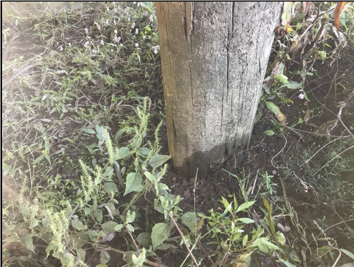
Bent 2 pile 4 minor decay at ground line.
