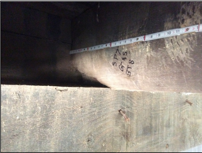
Span 7 girder 5 at bent 8, crushing.
