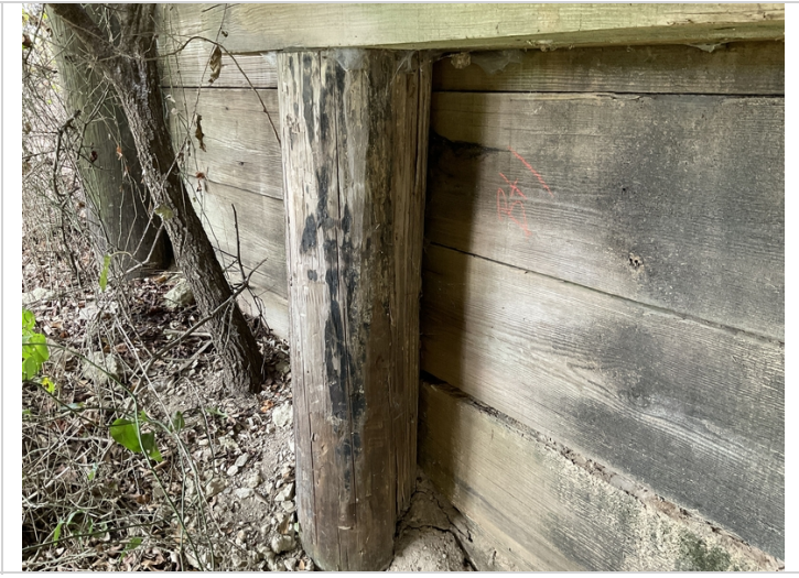
Bent 1 pile 4 split whole length
