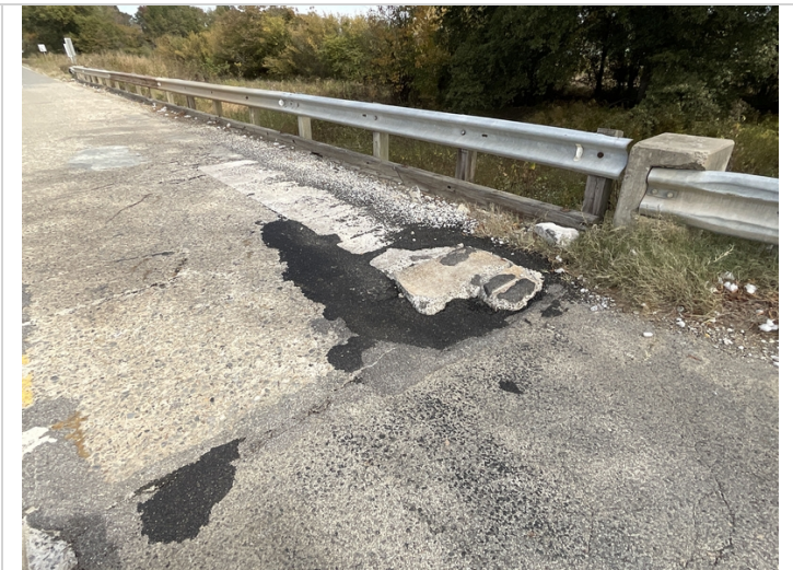
Patch in north bound lane has failed
