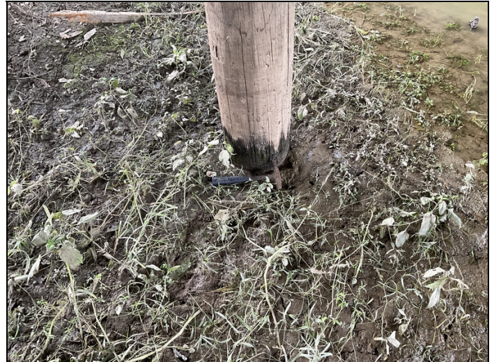
Bent 2 pile 2 has minor decay at ground line
