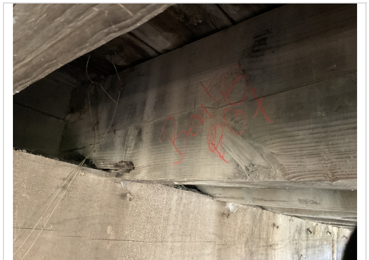
Bent 8 g7. bent 8 girders are decayed on the end
