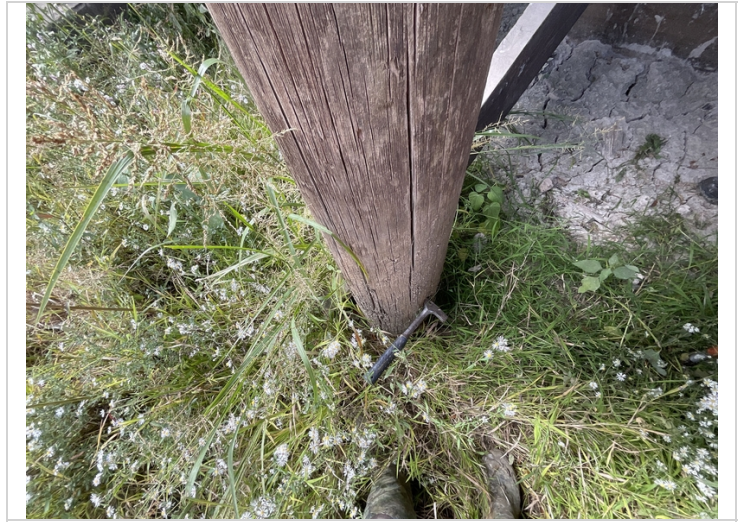
Bent 4 pile 1 is hollow at ground level
