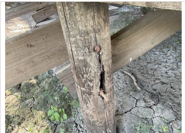
Bent 5 pile 2 backside is hollow around bolts
