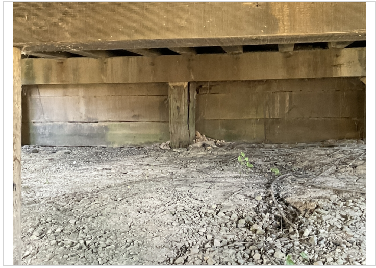
Bent 8 abutment pile 2 is split at the top and hollow
