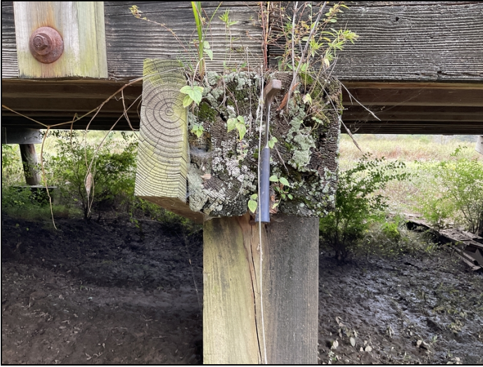
Bent 6 left end of cap is decayed 1'
