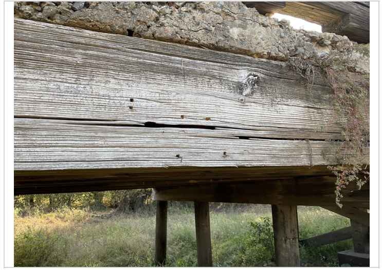
Span 2 girder 15 is hollow
