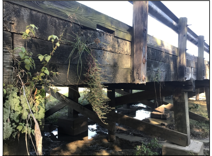
Span 5 girder 1, Typical outside girder condition
