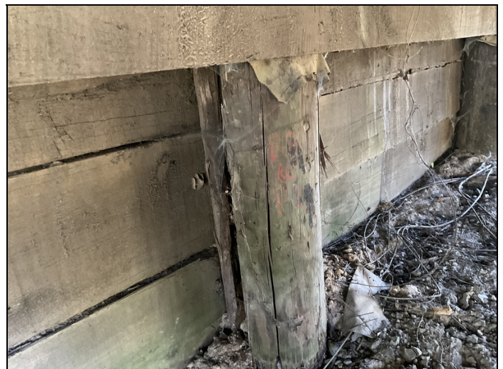
Bent 8 pile 2 is hollow and split 2022 picture
