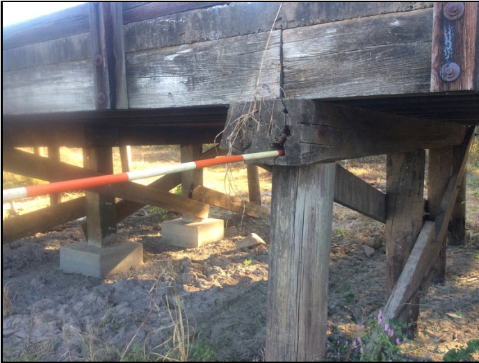
Bent 5 right end of cap decayed and hollow up to one foot.
