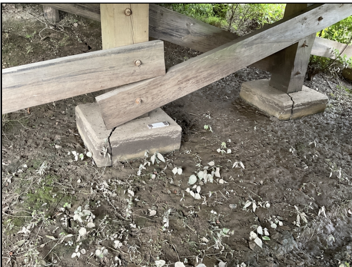
Bent 6, all concrete collars have large cracks.
