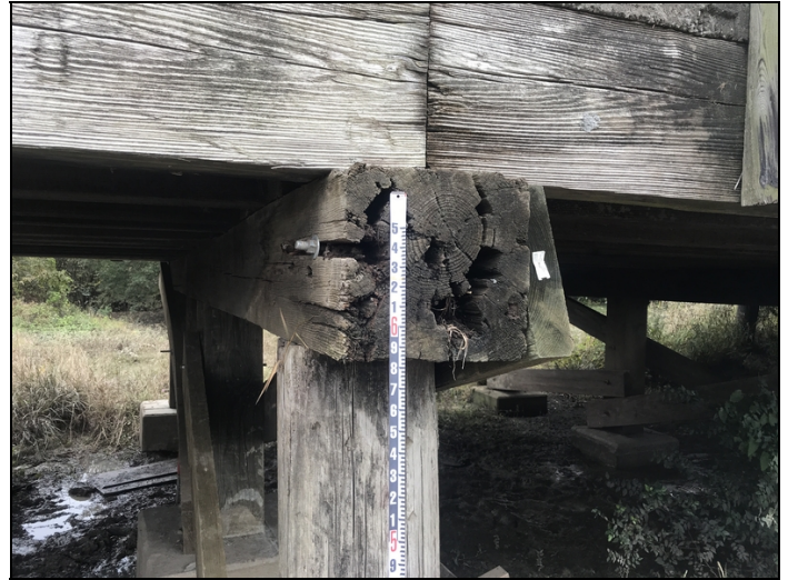
Bent 5: right end of cap is hollow
