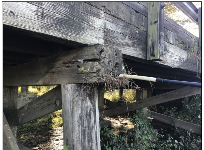
Bent 5 right end of cap is decayed and hollow up to 20"
