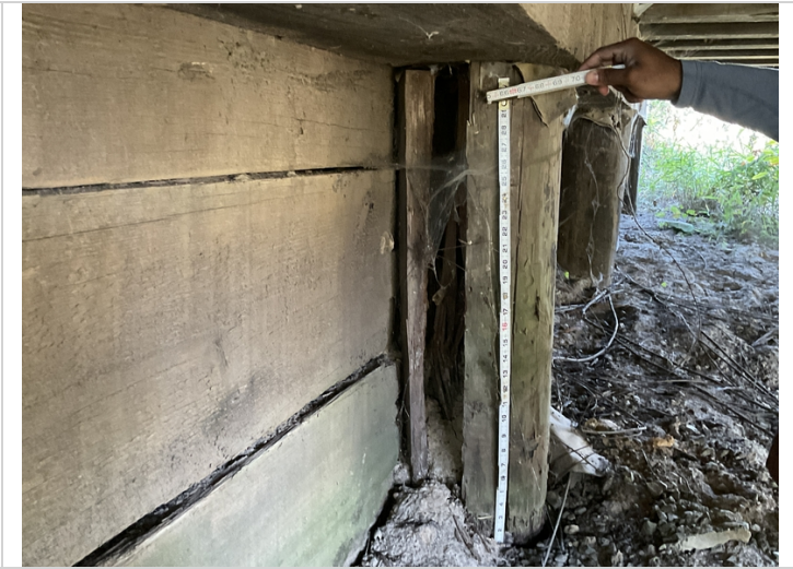
Bent 8 pile 2 is hollow and split 2022 picture
