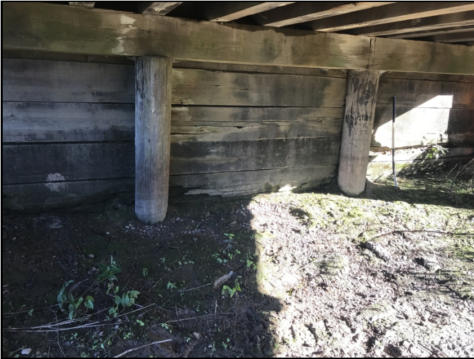
Timber cribbing at bent 1 is decayed.
