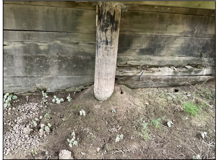
Timber cribbing at bent 1 is decayed.
