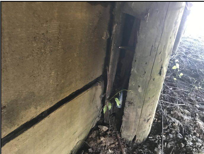
Bent 8 pile 2 hollow and decayed. Worst case this bridge.
