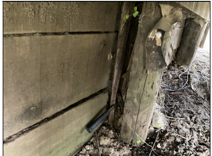
Bent 8 pile pile 2 is hollow and decayed (worst case this bridge)
