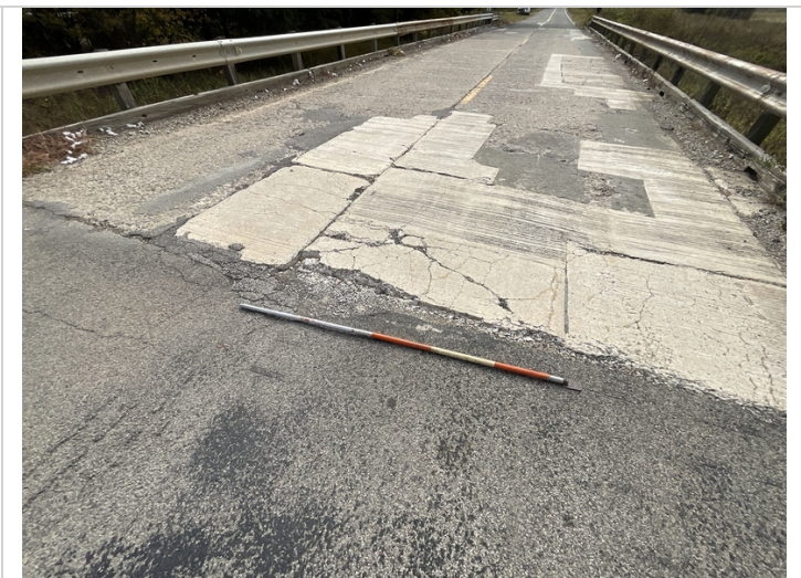
Large spall in the concrete at north end of the bridge
