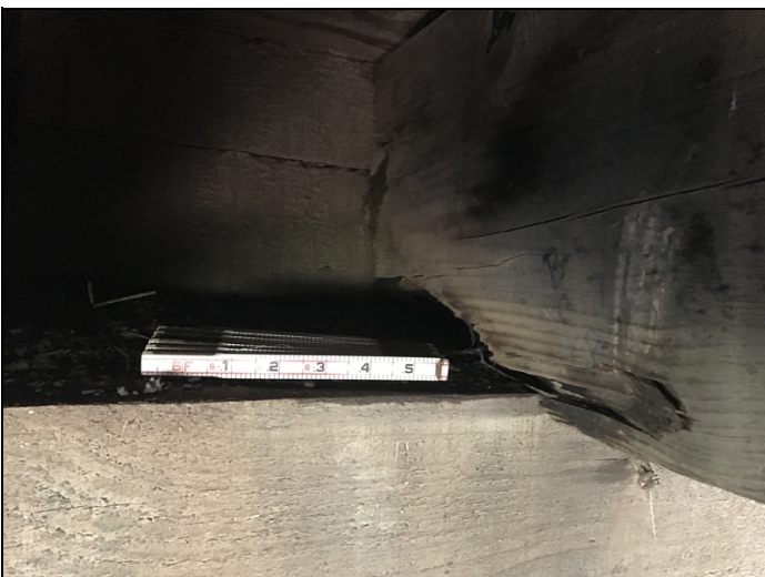
Girder 7 is decayed and crushing
