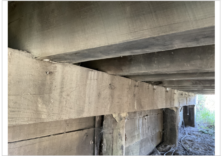
Bent 8 girder ends 2,3,4,5,6,7 and 8 are decayed
