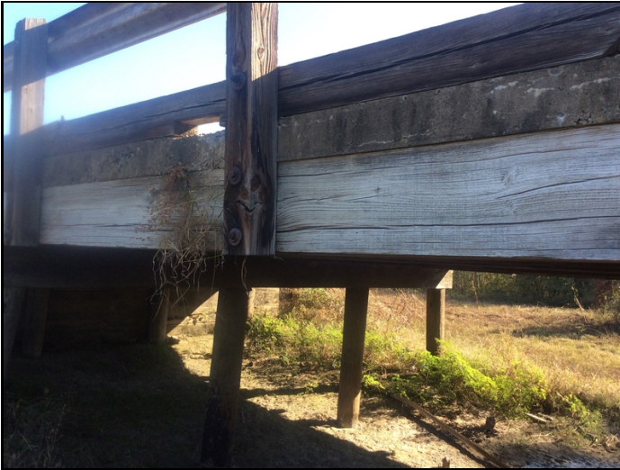
Span 2 girder 15 decayed and split.
