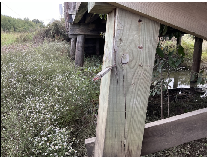
Bent 4, pile 4: wooden spliced pile that has a large split adjacent to the cap
