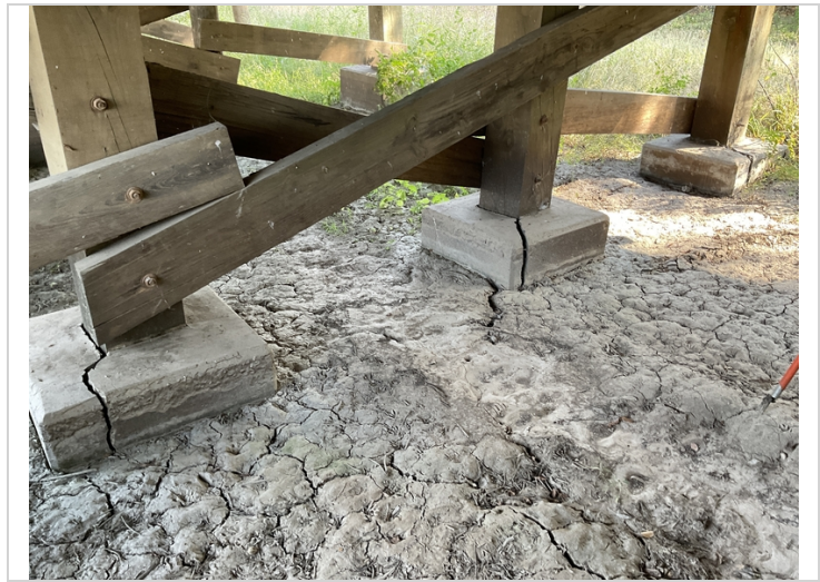
Concrete collars around the bottom of the pile at bent 6 have cracked and split
