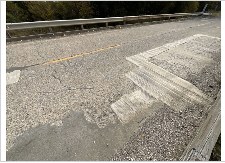
Large cracks and patch areas
