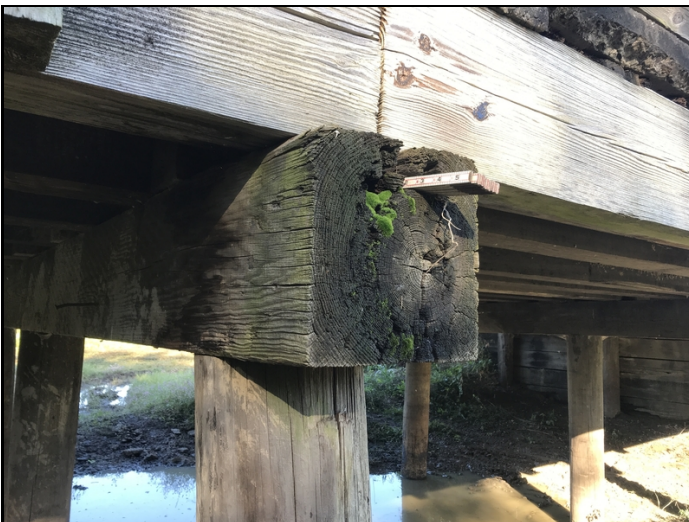
Bent 3 left side of cap is decayed.
