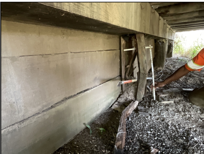
Bent 8 pile 2 has failed and is crushed
