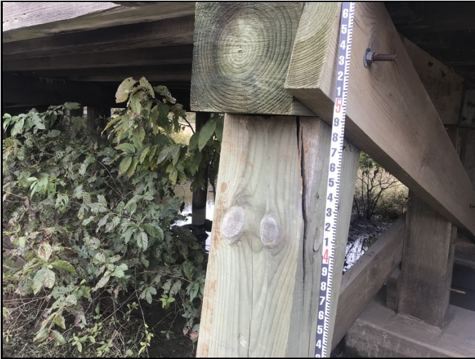
Bent 4, pile 4: this is a newly placed wooden spliced pile that has a large split adjacent to the cap
