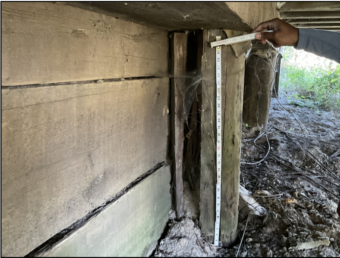
Bent 8 pile 2 is hollow and split 2022 picture
