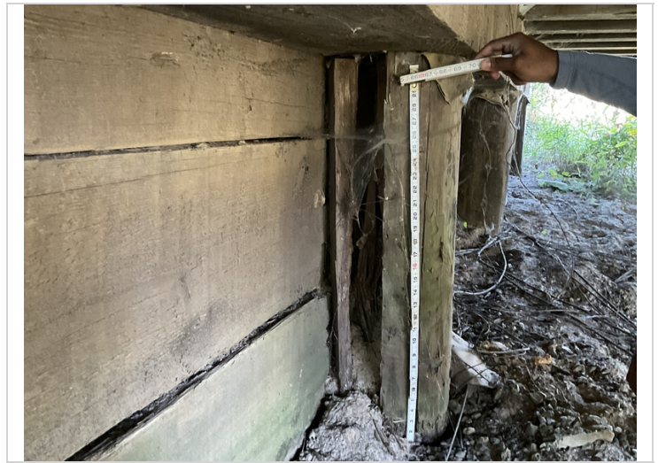
Bent 8 pile 2 is hollow and split 2022 picture
