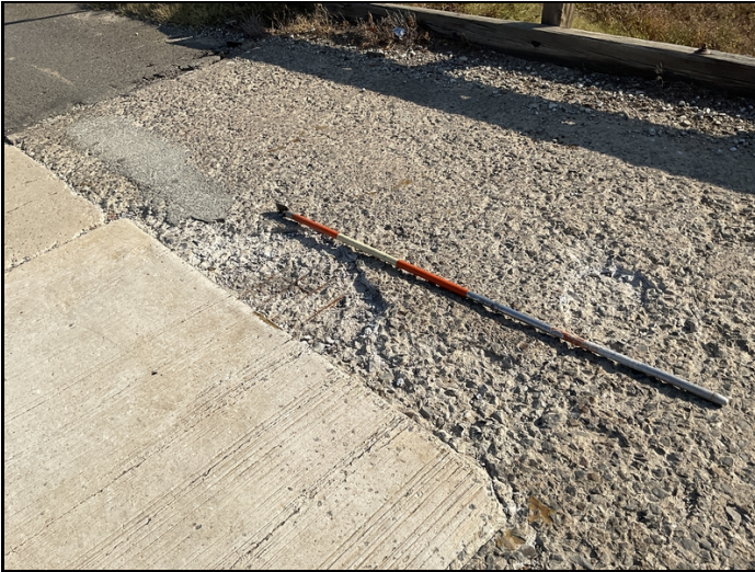
Large spalls with rebar exposed in span 1
