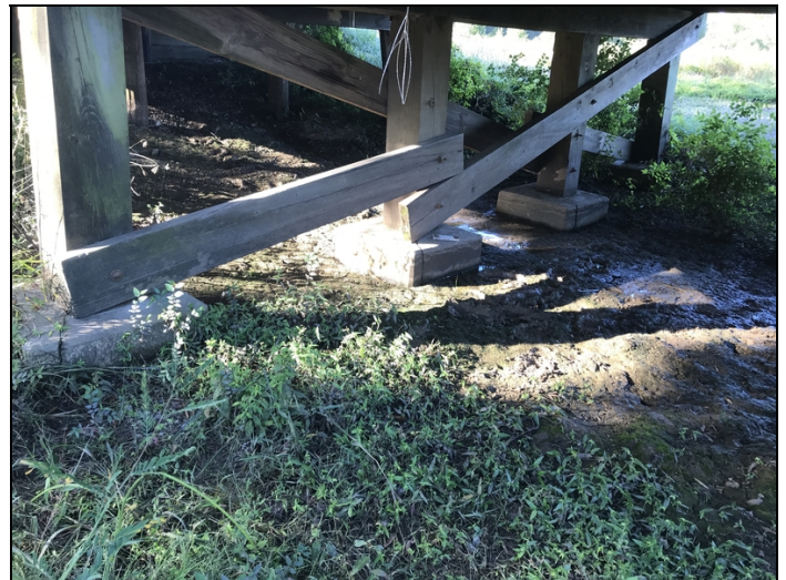
Bent 6, all concrete collars have large cracks.
