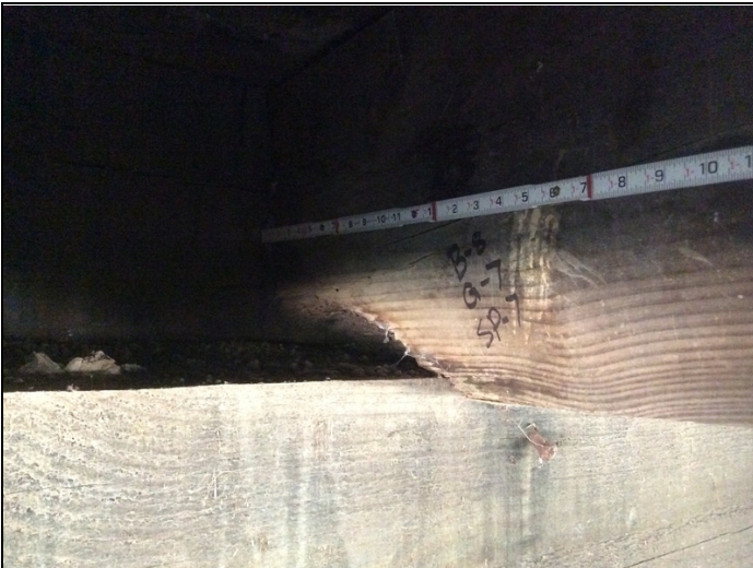
Span 7, girder 7 at bent 8, crushing.
