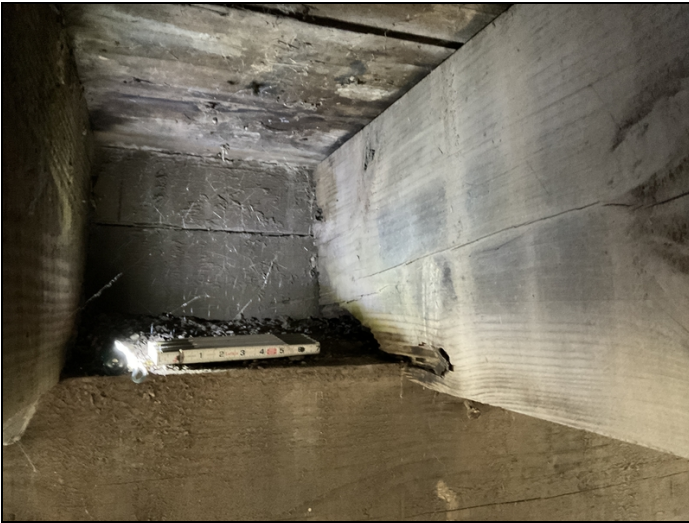
Span 7 girder 8 at bent 8, decayed and crushing
