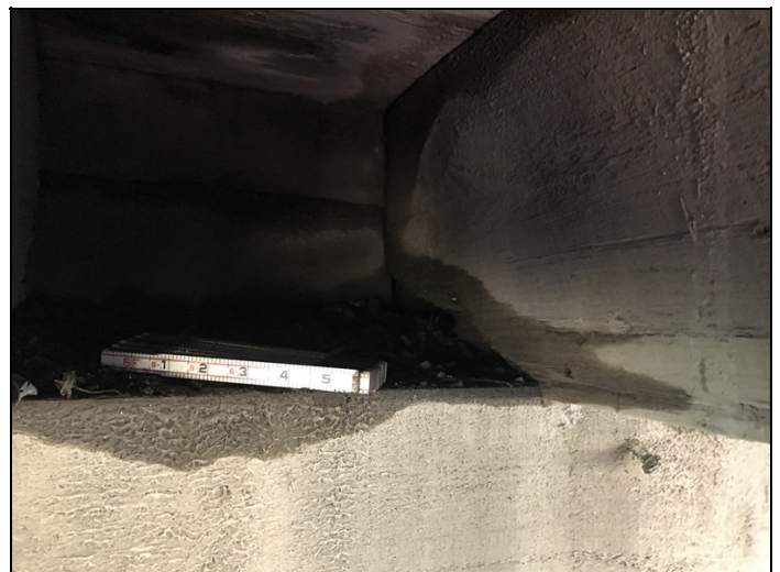
Girder 8 is decayed and crushing
