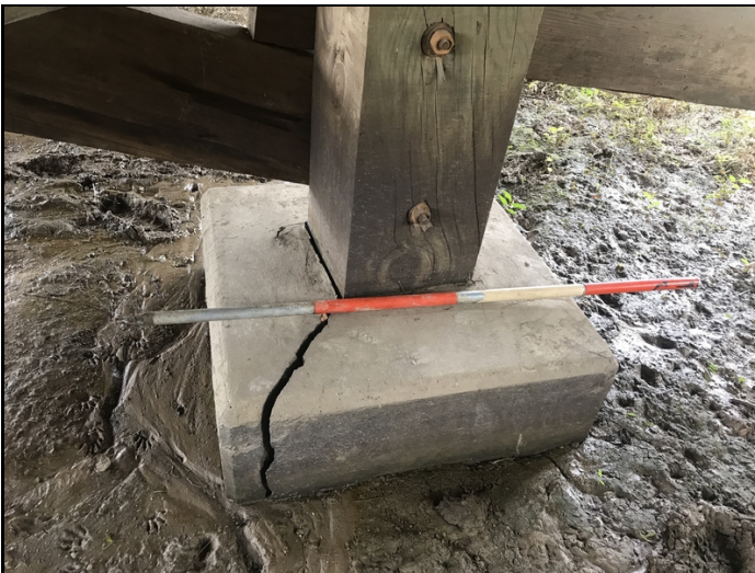
Bent 6, pile 2: concrete collar with large crack. Similar condition at pile 1 at this bent
