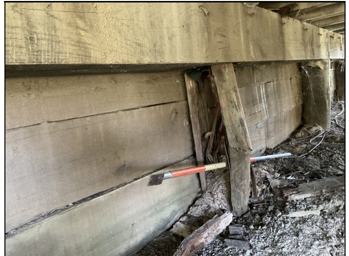
Bent 8 pile 2 has failed and is crushed
