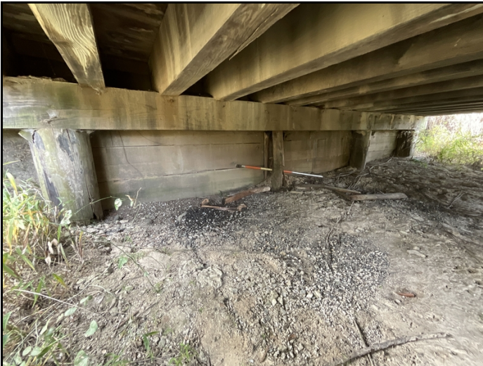
Bent 8 pile 2 has failed and is crushed
