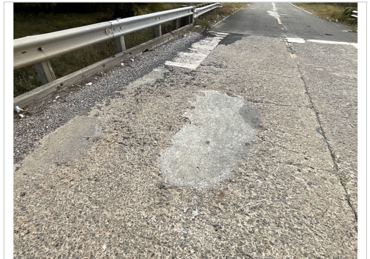
Heavy scaling in north bound lanes
