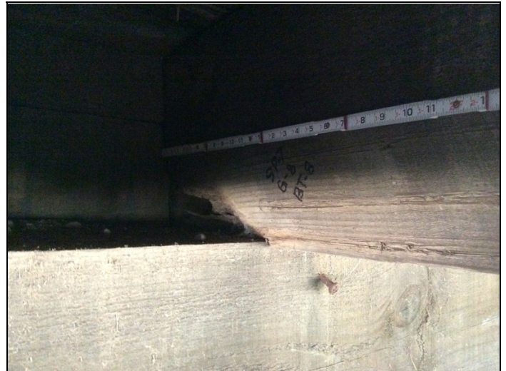
Span 7, girder 8 at bent 8, crushing.
