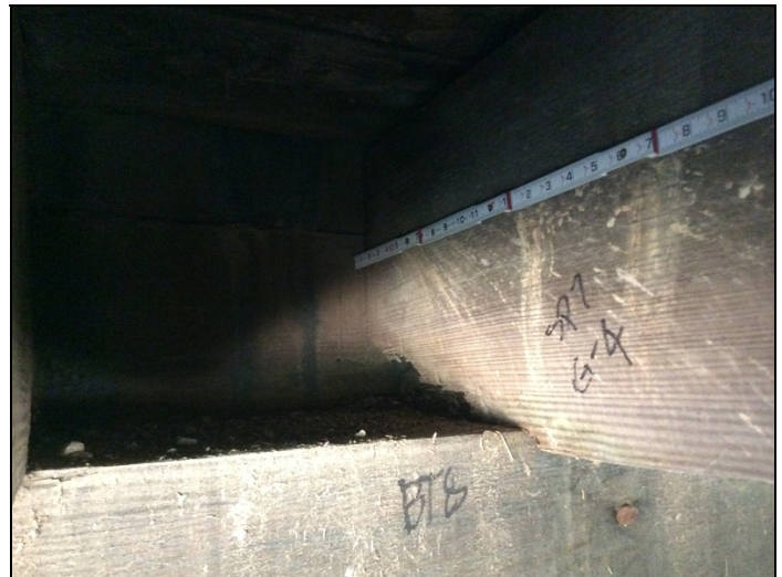
Span 7 girder 4, crushing at bent 8
