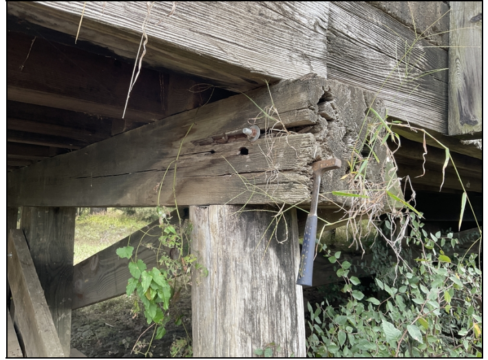
Bent 5 right end of cap is decayed up to 20"
